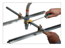
Verify that the reducer is located in the correct intended position before securing the bracket. Check and adjust the reducer position by moving vertically and horizontally along the square Bar. The distance in between the end of spiral of reducer and the side of bracket (L) shall keep over than minimum 20mm [Bracket (L) torque: 65Kg.cm] when assemble the reducer through the bracket (L). Tighten all the bolts securely and evenly.
